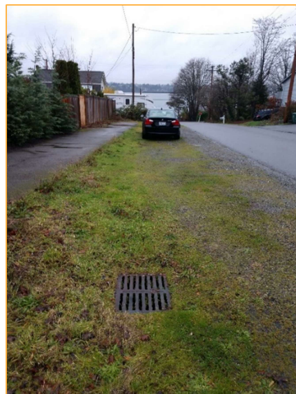
Photo N6 – Facing west along SE 28 th St approximately 150 feet west of Photo N5. Runoff is conveyed via this catch basin on the south side of the street toward Lake Washington.
