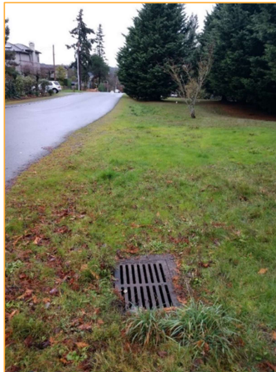
Photo S1 – Facing west along the north side of SE 30 th St. Onsite runoff sheet flows in the southwestern direction to the catch basin above and is conveyed west toward Lake Washington.
