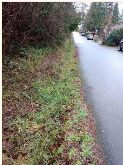
Photo S4 – Facing south on the east side of 62 nd Ave SE approximately 60 feet from Photo N4. Onsite runoff sheet flows in the southwest direction toward the ditch above and is conveyed south to be combined with the south basin downstream conveyance system.
