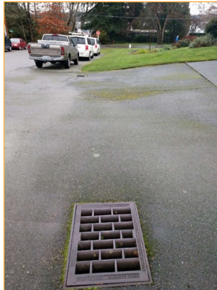
Photo S10 – Facing west along the north side of SE 30 th St approximately 30 feet west of Photo S9. Runoff is conveyed west toward Lake Washington.
